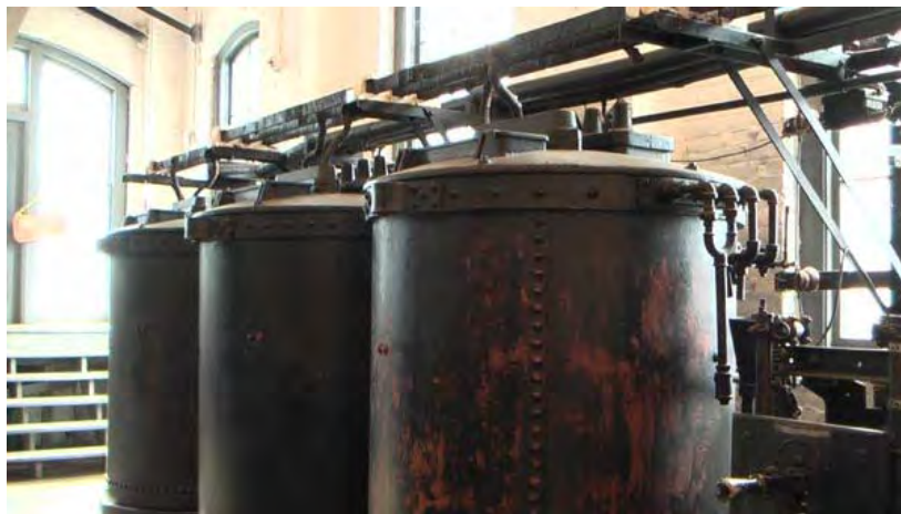
Westinghouse Transformator aus 1917 Hydropower plant Folsom, California.
